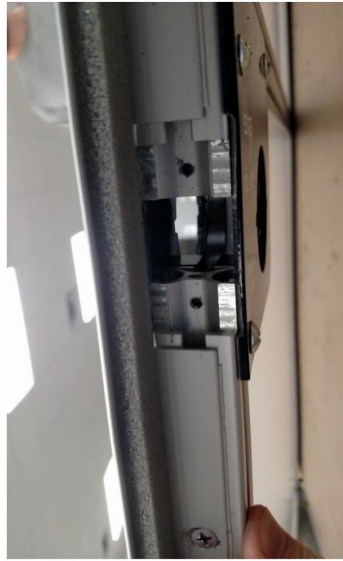
Standard Lever Style Lock – Supplied with our doors. Keyed on the outside pushbutton inside. Normally they are used with a classroom function but can be changed to storeroom.
